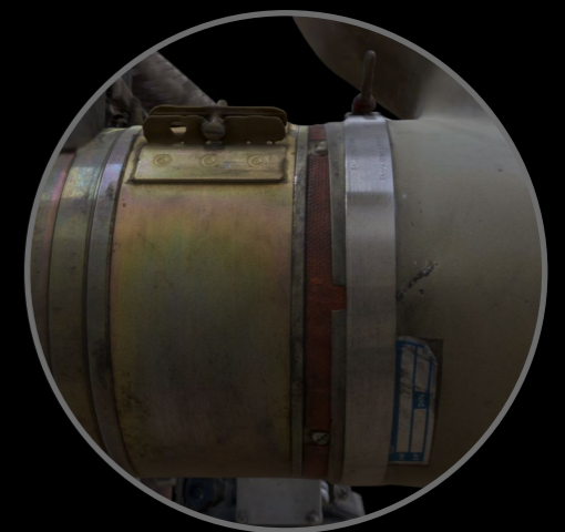
E. Damage and surface defects
